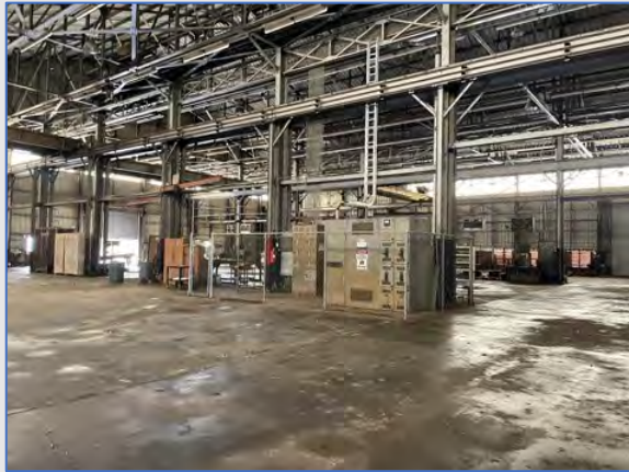
Maintenance shop interior
