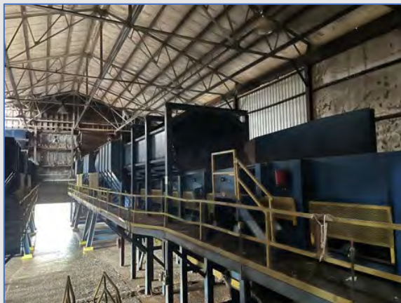
Main Plant Interior
