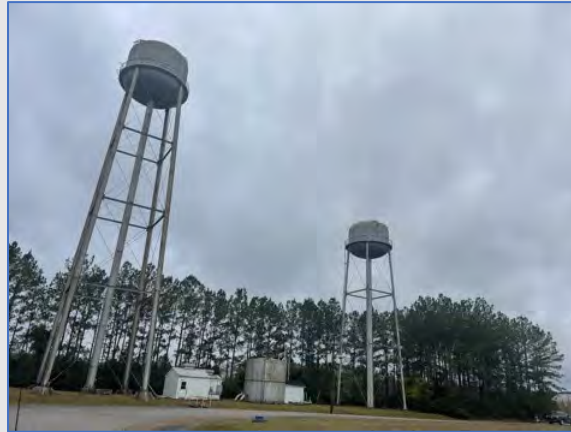
On site water supply
