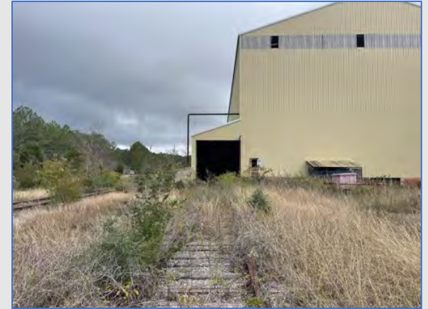
Rail access to main plant
